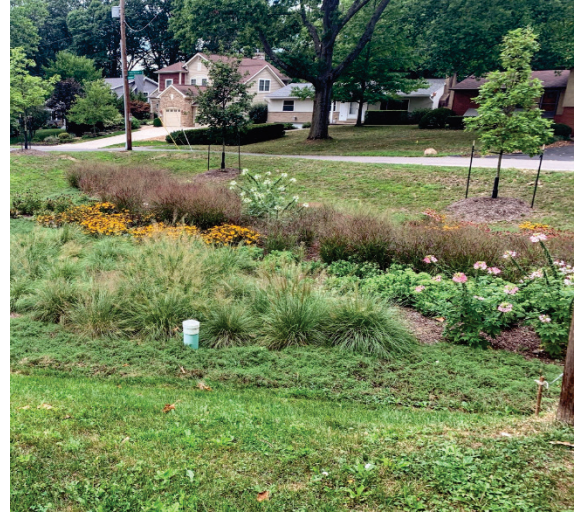
Completed regional bioretention basin.
