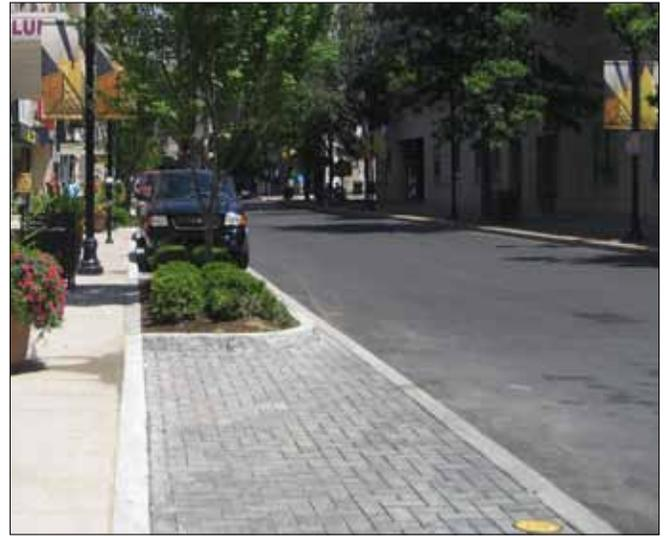
**RAIN GARDENS (bump outs and planters):** Larger planting areas that are sized to allow for stormwater infiltration and storage. Can be located in bump outs, in sidewalk planters, or as swales in existing tree lawns.
