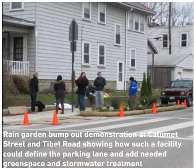
Rain garden bump out demonstration at Calumet Street and Tibet Road showing how such a facility could define the parking lane and add needed greenspace and stormwater treatment
