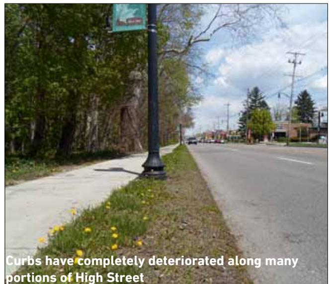
**Curbs have completely deteriorated along many portions of High Street**
