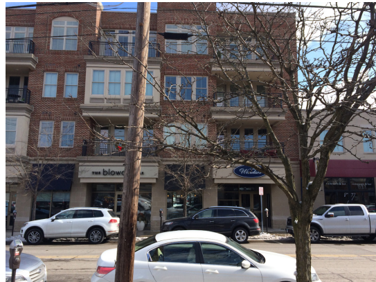
FOUR STORY WITH ADJOINING TWO STORY
