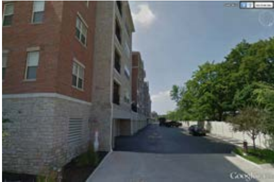
ARLINGTON CROSSING EXTERIOR PARKING
