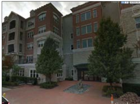
ARLINGTON CROSSING MAIN ENTRY
