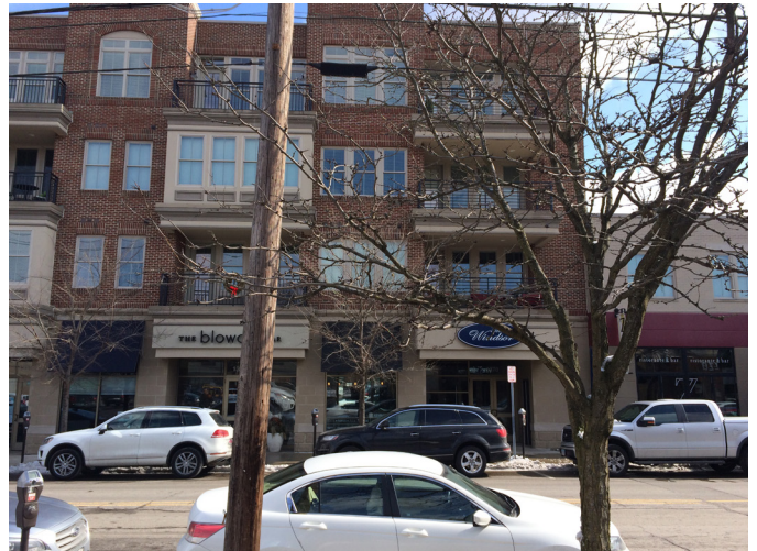
FOUR STORY WITH ADJOINING TWO STORY
