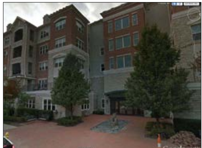
ARLINGTON CROSSING MAIN ENTRY
