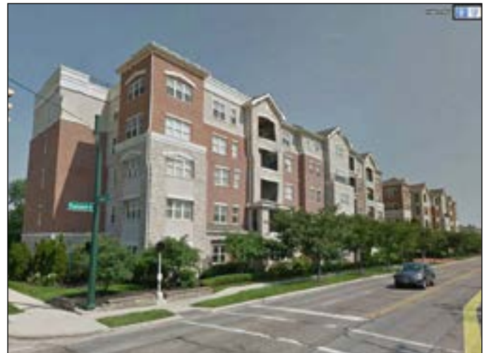
ARLINGTON CROSSING STREETVIEW
